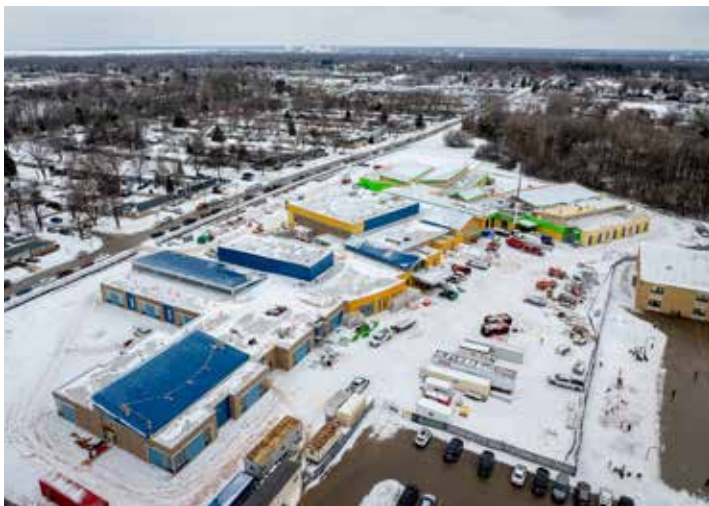
Newly constructed Starr Elementary incorporates geothermal and solar to meet district goals. Photo credit: GBAPS
