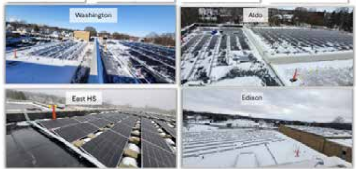
Solar panels installed on GBAPS schools including Washington and Edison Middle Schools, Aldo Leopold Community School, and East High School. Photo credit: GBAPS
