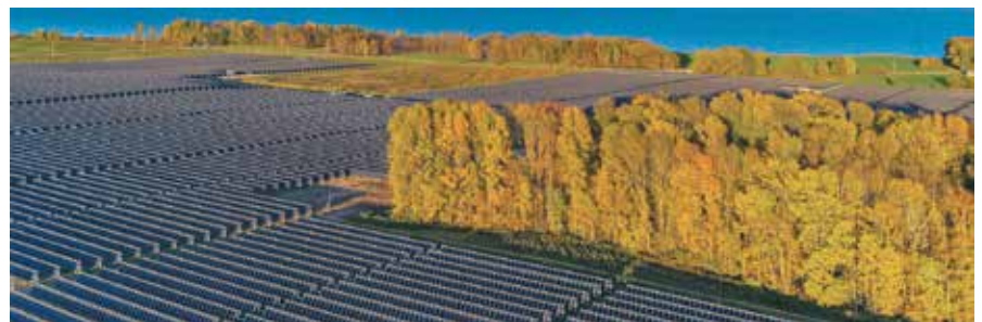
Two Creeks Solar Park. Photo credit: Wisconsin Public Service
